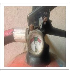
02 out of 6 fire extinguishers located on ground floor found with low pressure level.
